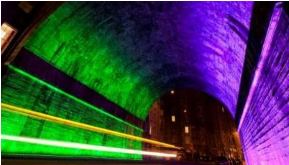
The Regent Bridge Edinburgh, UK
